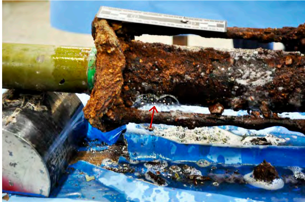
Figure 20: Another view of the leaking location, arrow.
