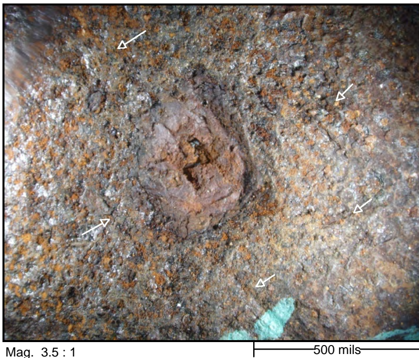
Figure 64: Failed location at 4 o'clock: An overall view of the corroded spot on OD. Arrows point to parallel line type surface impression around the corroded spot. Another view.
